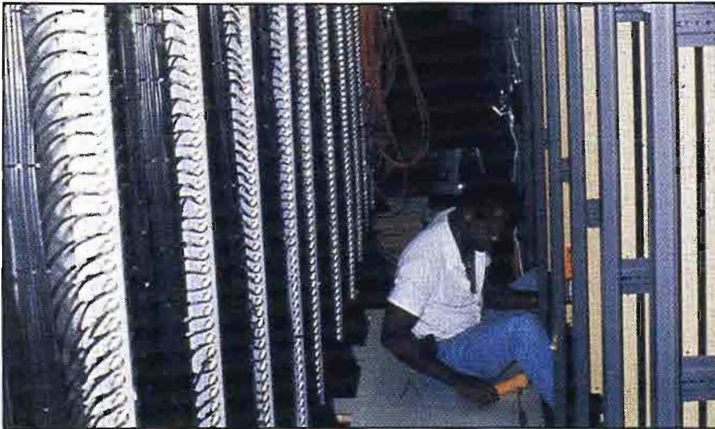
One of the 40-foot containers equipped with communications systems, audio and video patching and distribution matrices.
